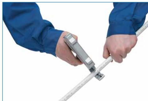
Cut the pipe perpendicular to its axis using special cutter.
