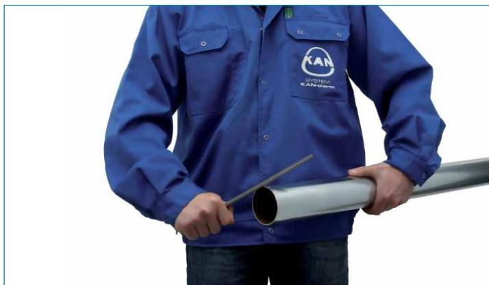
**3. Marking the insertion depth of the pipe in the fitting**
