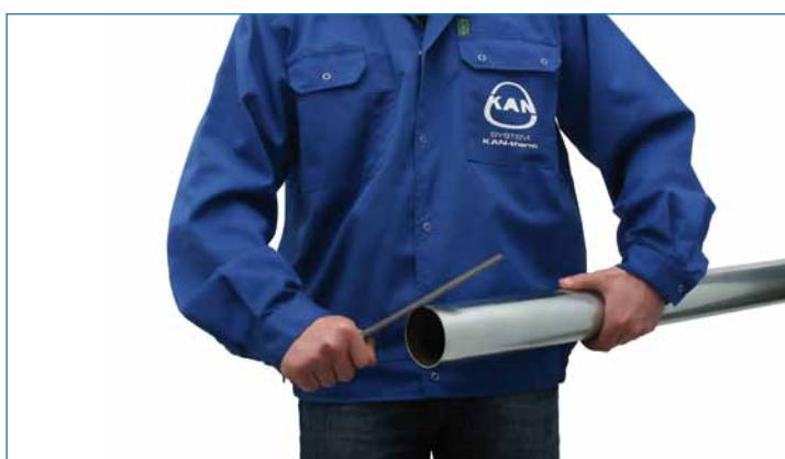
**3. Marking the insertion depth of the pipe into the fitting**
