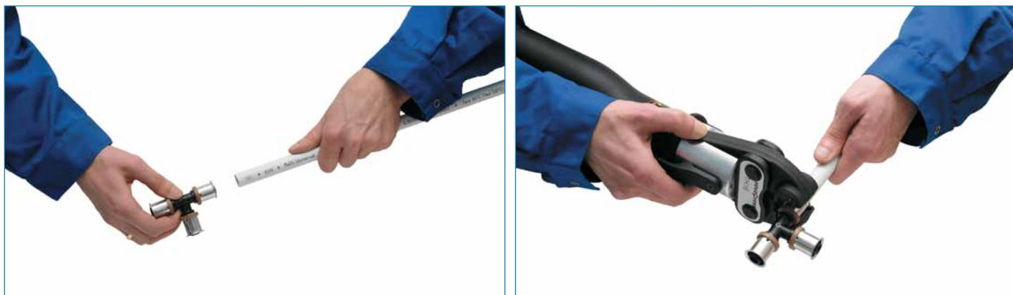
3. Insert the pipe into a coupling - push the pipe centrally along the coupling axis. Check the insertion depth - the pipe edge must be visible in inspection holes in the steel ring.
