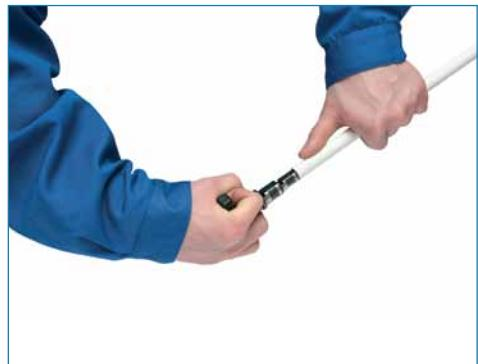
Cut the pipe perpendicular to its axis using special cutter.
