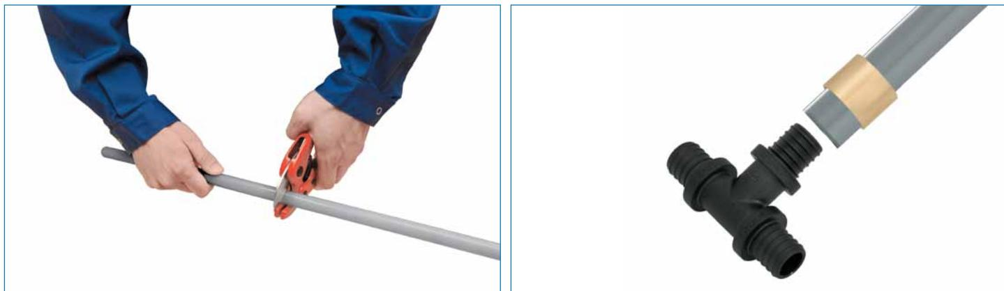
1. Cut a multi-layer PE-Xc/Al/PE-HD Platinum pipe to a required length with scissors. The cut must be perpendicular to the pipe axis.
