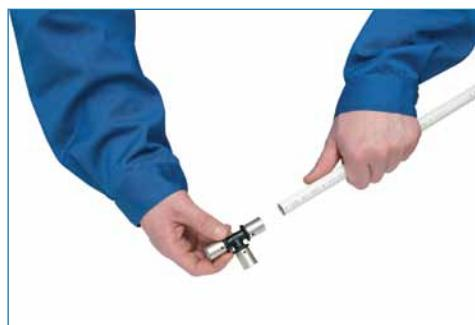
Through inspection holes in the steel ring check if a pipe is inserted right – it must be visible in the holes
