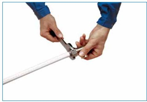
Insert the screwed joint body into a pipe till it definitely stops. The joint insertion depth is ca. 9 mm for pipes Ø14, 16, 20 and 12 mm for pipes Ø25, 26.
